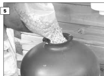
Fill the filter first with gravel (3-5mm) and then with sand (0.4-0.8mm). The sand has an unlimited lifetime and only need to be topped up in case sand is lost. Mark the level of sand/gravel to be able to re-fill the filter to the correct level at a later time.
