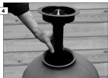
Make sure that the plastic protection (funnel) is placed on top of the filter to prevent sand/gravel from falling into the mouthpiece of the branch pipe.
