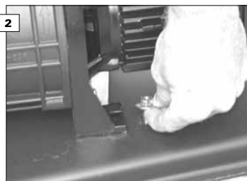
Attach the pump to the pedestal with the enclosed bolts (+nuts and washers).
