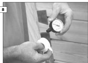
Now apply Teflon tape to the outer thread of the manometer.
