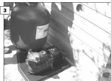
Place the filter on the pedestal and fill it with a 1/3rd water.
